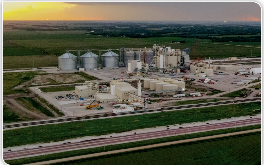
AGP’s new processing facility in David City, Nebraska, can process more than 50 million bushels of soybeans annually.
