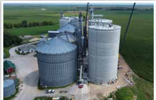
Manning Rail and Manning Grain in Burress, Nebraska, an unincorporated community in Fillmore County.
